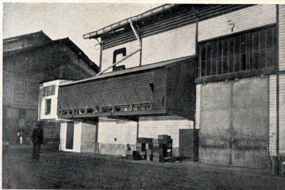
INSTALLATION FOR UNLOADING BAGS IN THE QUAY.
